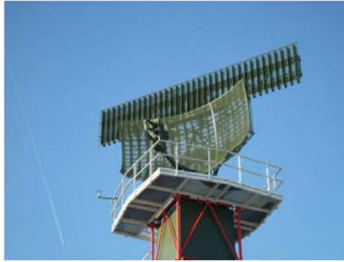
Secondary Surveillance Radar Antenna
